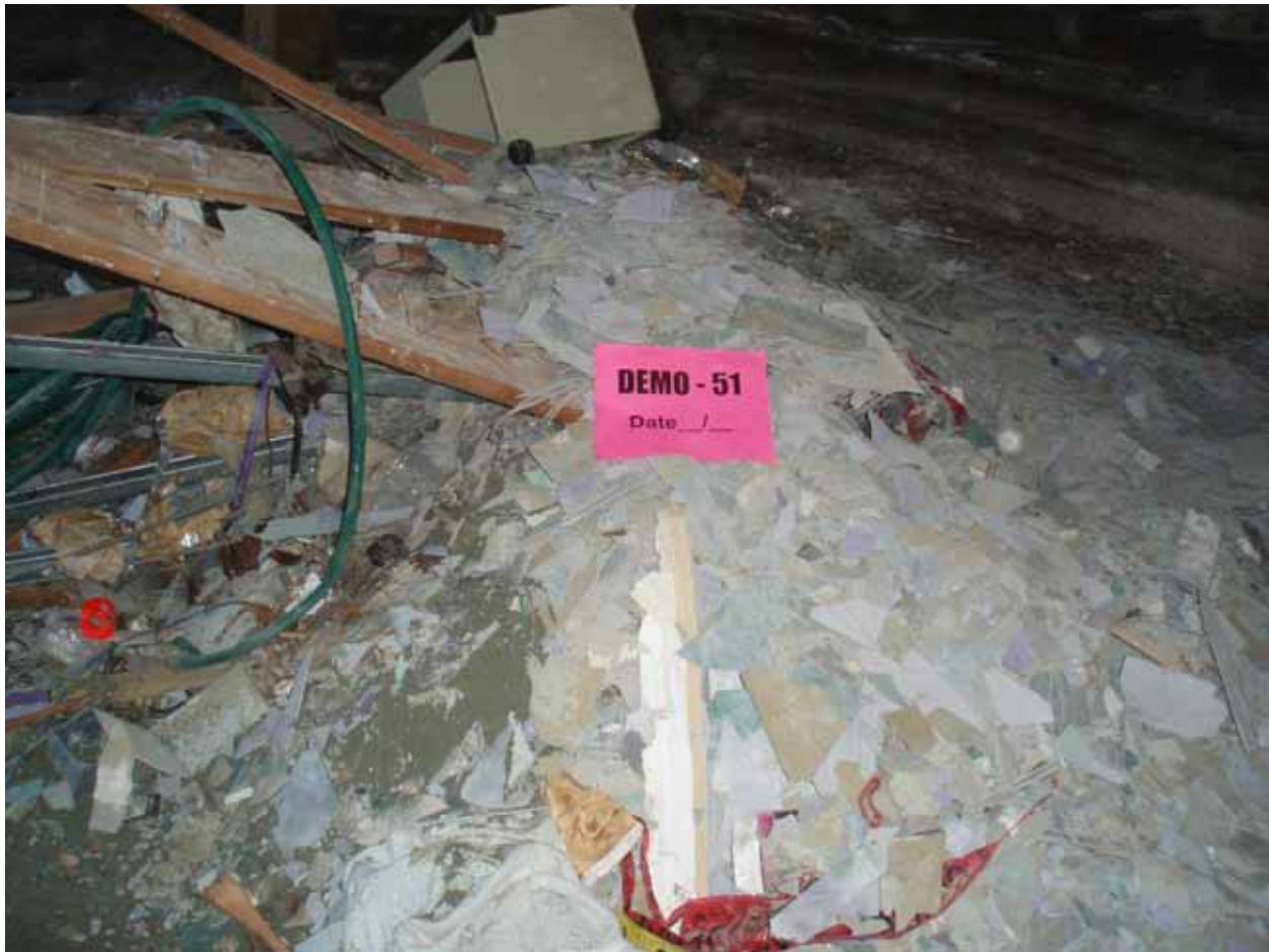
Figure H-4. Other Aggregates in Transfer Station Disposed Sample Number DEMO-51
