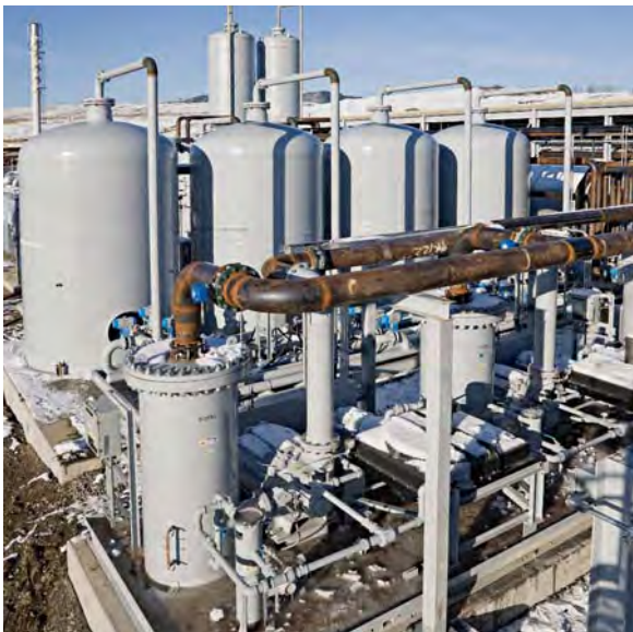
Components will "clean" the landfill gas to ready it for the energy grid.
