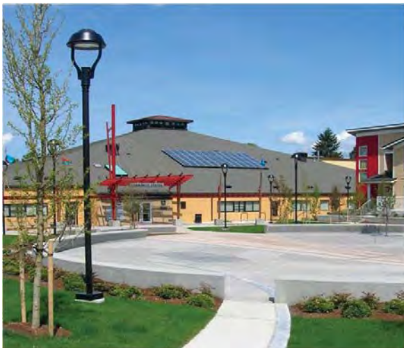
Renovation of the award-winning Jim Wiley Community Center in White Center saved energy and resources by recycling the previous building at the site rather than demolishing it and starting anew.
