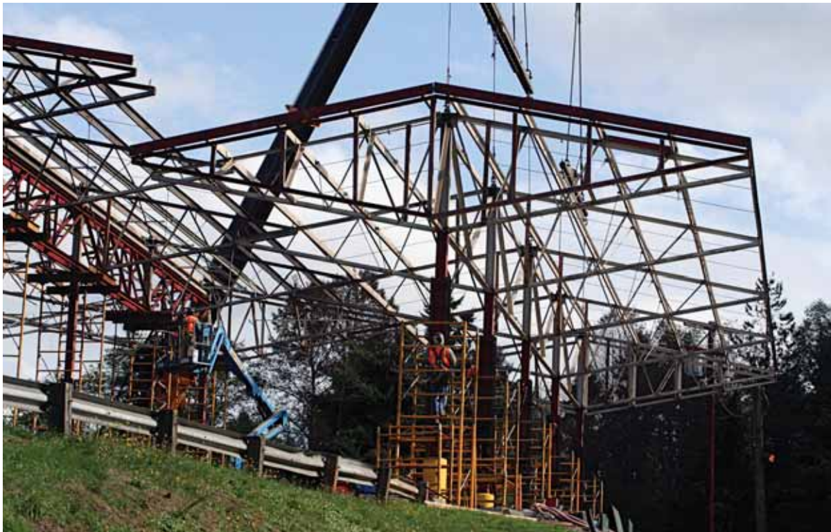
The roof at Houghton Transfer Station was raised in four sections.
