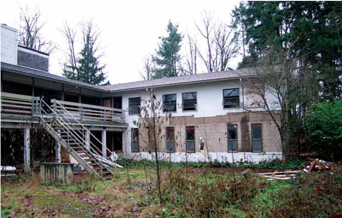
Fagan Hall, a 14,000 square foot dormitory at the former Cedar Hills Alcohol Treatment Facility before deconstruction.
