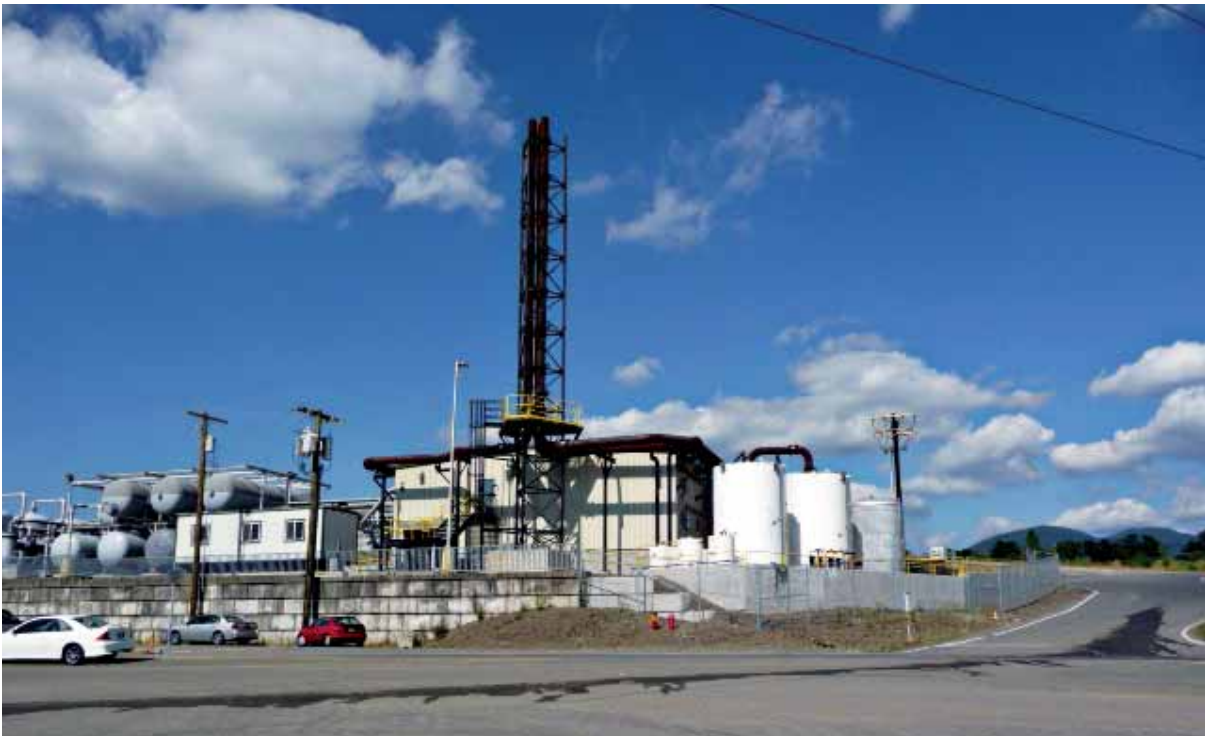
BEW refines landfill gas into pipeline quality natural gas, bringing revenue into the division.
