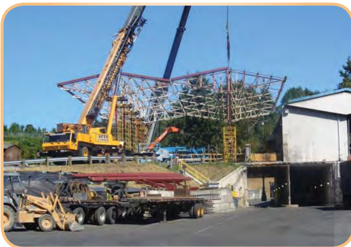
The roof at Houghton Transfer Station was raised to allow commercial trucks to operate more safely.
