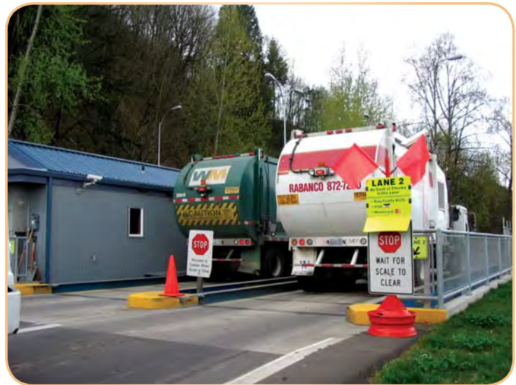
The use of two outbound scales at the Algona Transfer Station allows the station to continue operating above its designed capacity, but has not eliminated congestion.
