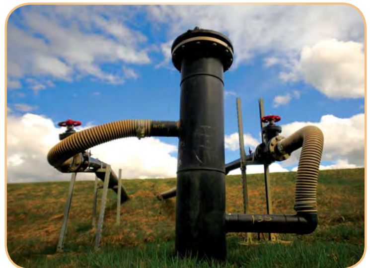
An extraction well collects gas from the landfill and routes it to the landfill gas-to-energy facility for conversion to marketable natural gas.
