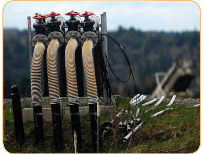
Collecting landfill gas as the garbage decomposes over time is a crucial element of pre- and post-closure maintenance.
