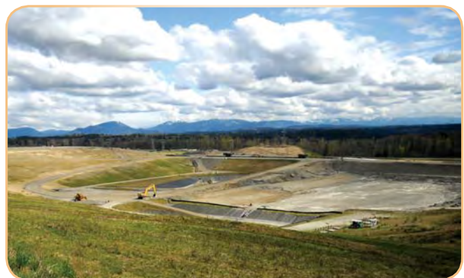
The landfill has been developed in sequential stages (or refuse areas), most recently with construction of Area 7.
