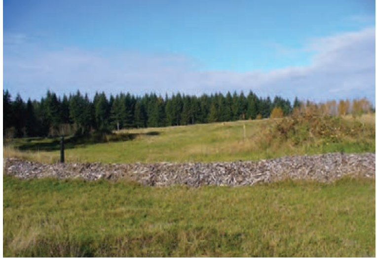
A bioherm at the Cedar Falls closed landfill filters landfill gas.
