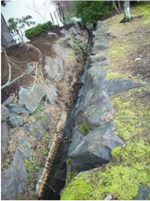
Photo 21. Ditch A facing north – the channel lined with a half-cut CMP
