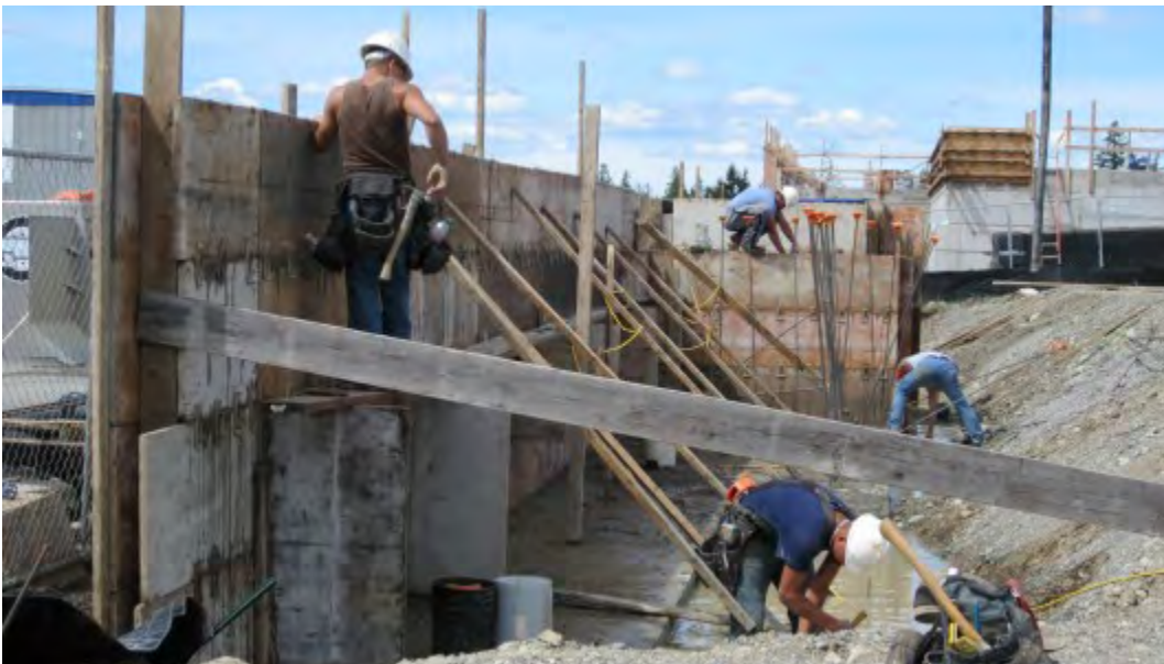
zHome retaining wall under construction
