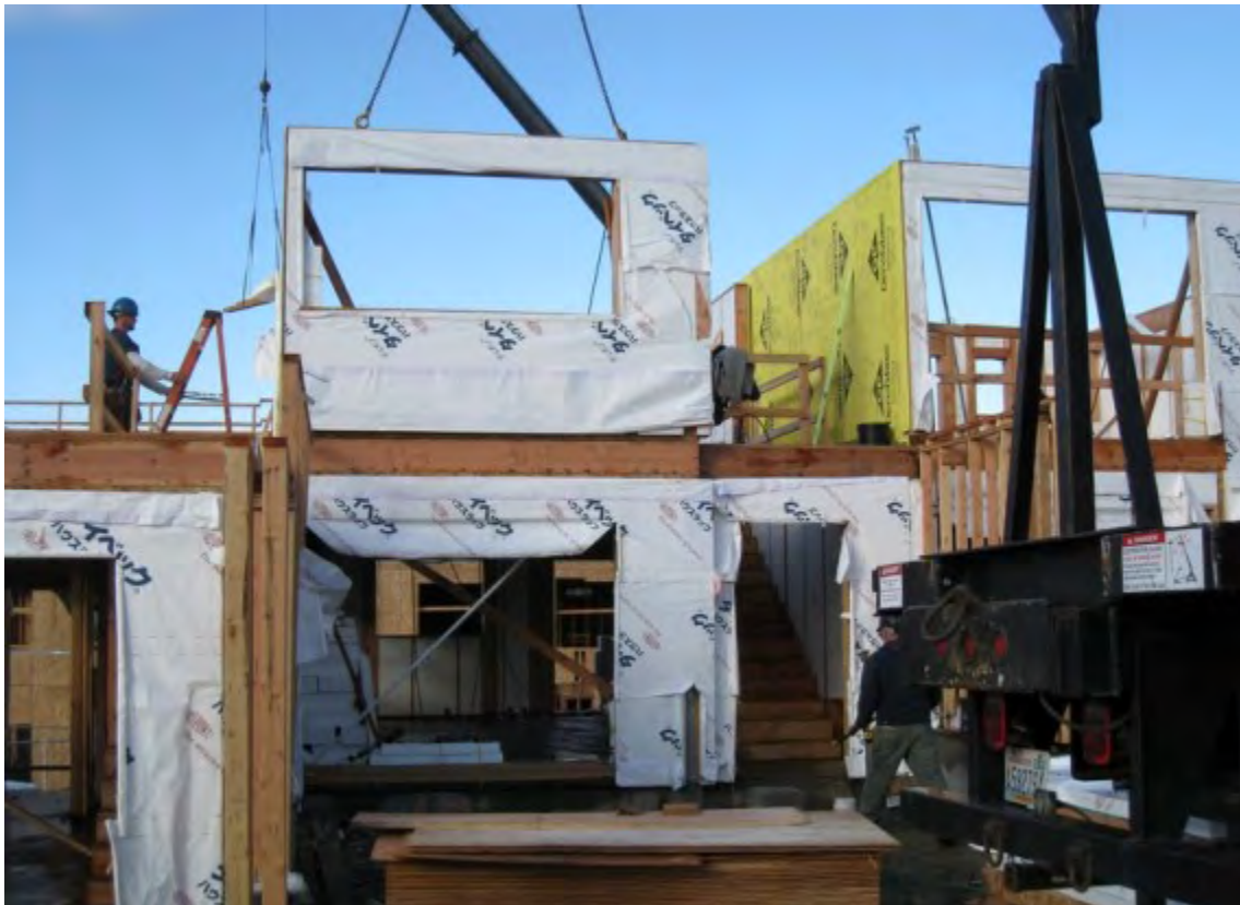
Panel being dropped into place
