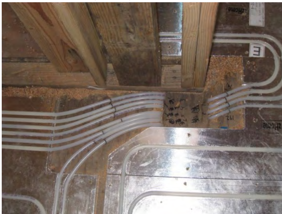
Hydronic heat pipes coming up through one floor to the next
