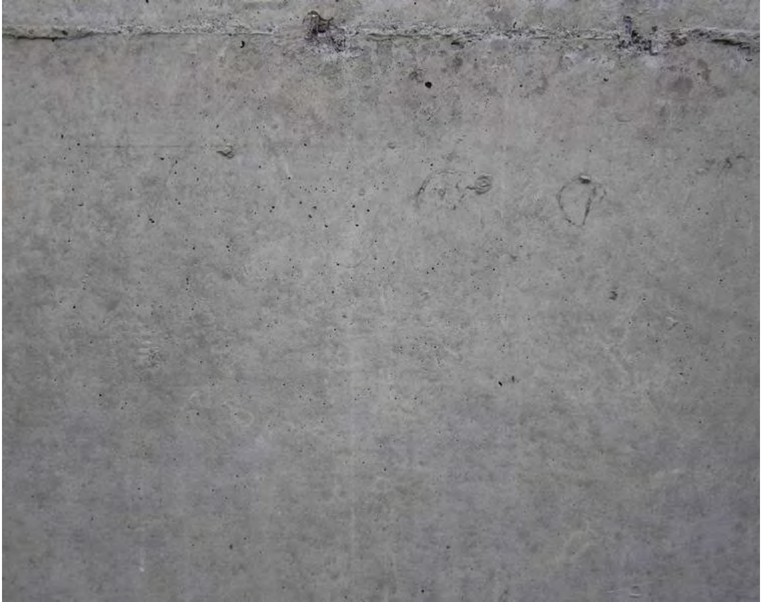
Closeup of 30% flyash wall - almost void free.
