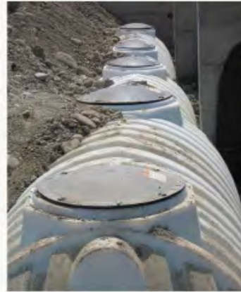
1,700 gallon cisterns for units 4-6. Units 1 and 2 have 1,000 gallon cisterns which sit partially above ground, and units 3-10 have 1,700 gallon cisterns which are completely buried.
