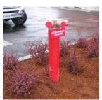
department supplies water to the fire protection standpipe or sprinkler system.
