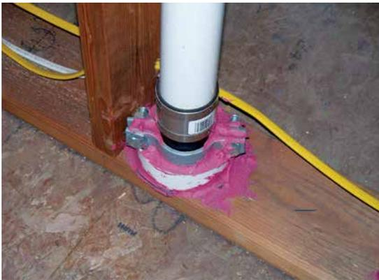
*In a kitchen or bathroom remodel, or new construction, sealing plumbing penetrations is easy and effective. Source: O'Brien & Company*
