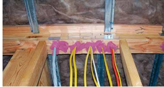
*In an addition, new construction or a gut remodel, there are many opportunities to seal electrical penetrations and top and bottom plates. Source: O'Brien & Company*
