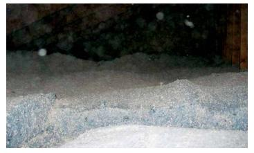
Any attic insulation should be smooth across the entire home. Mounding, lumps, valleys, voids and other problems with uniformity significantly reduce the overall R-value of the insulation. Source: O'Brien & Company.
