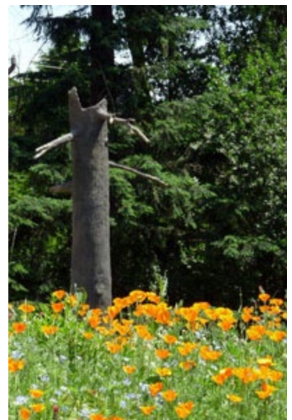
The only above ground structure in Boeing Creek Park is an odor control stack disguised as a tree snag.
