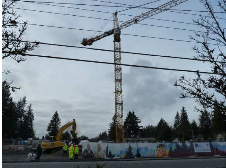
Under construction as of January 2019
