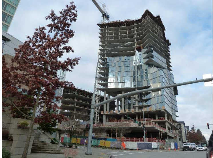
Under construction as of January 2019
