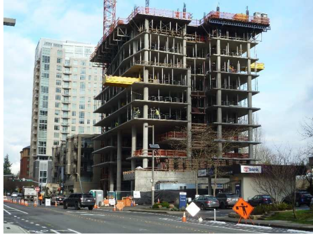
Under construction as of January 2019
