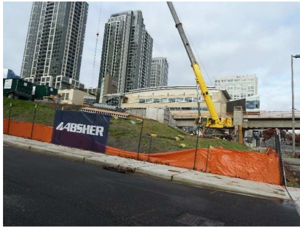
Under construction as of January 2019
