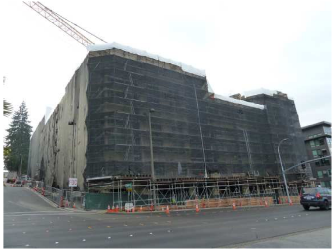
Under construction as of January 2019
