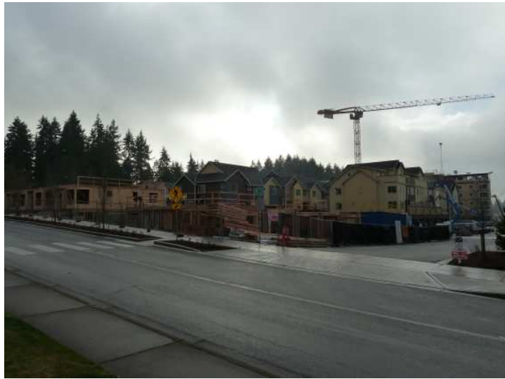
Under construction as of January 2019
