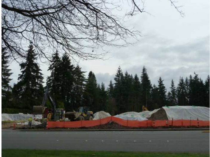
Under construction as of January 2019
