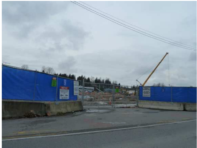
Under construction as of January 2019
