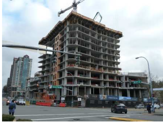
Under construction as of January 2019
