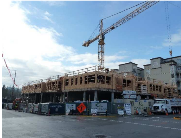
Under construction as of January 2019
