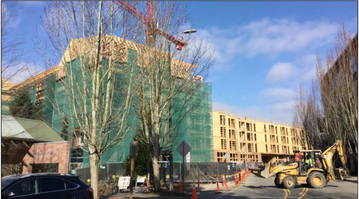
153 unit apartments & YMCA project #159940-0050
