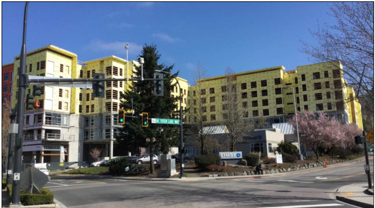
Upper Totem Lake Mall under construction #894439-0010
