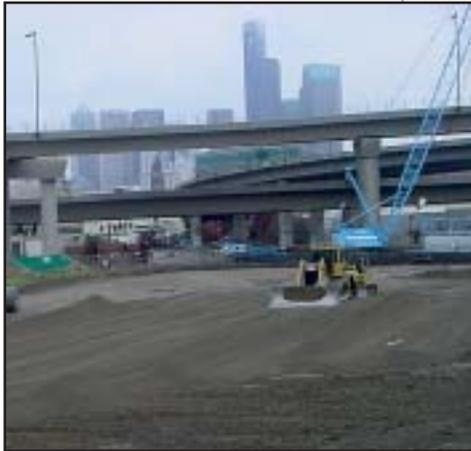
*"The crushed concrete readily achieved specified compaction criteria for use as select backfill for construction of a 5-story parking garage."*
