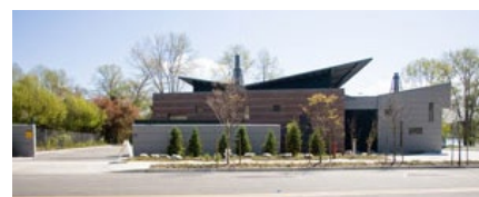
New Juanita Bay Pump Station, on the corner of Northeast Juanita Drive and 93rd Avenue Northeast, April 2009
