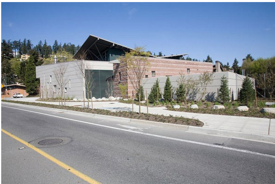
Juanita Bay Pump Station
