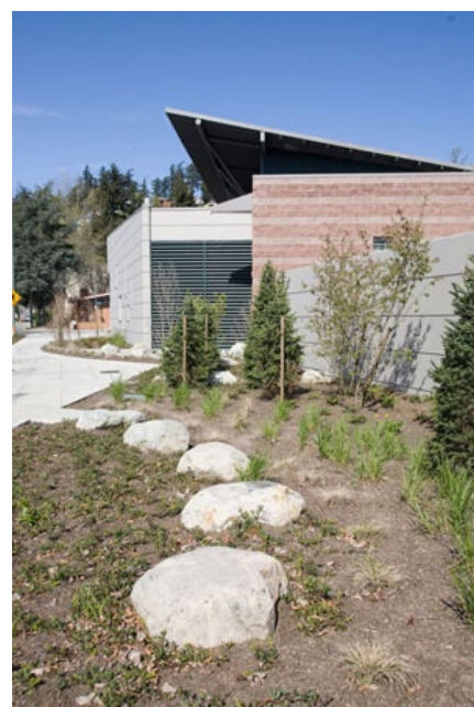
Pump station landscaping, southwest corner
