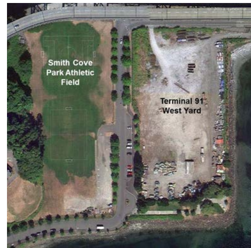
Smith Cove Park/Terminal 91 West Yard area today. King County's project will use space in both areas for construction.
