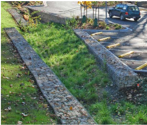
Gabion walls, a landscaping element that will be used to evoke the storage tank bays underneath the surface (see C on the diagram at right).
