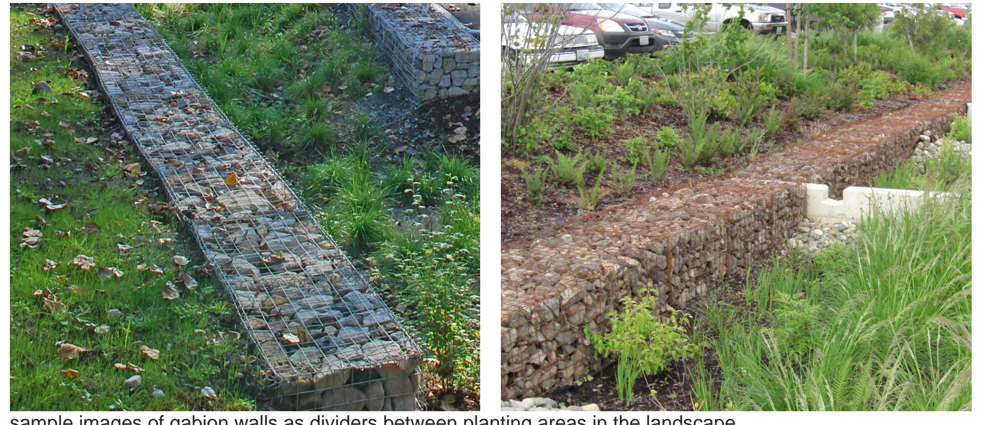
sample images of gabion walls as dividers between planting areas in the landscape
