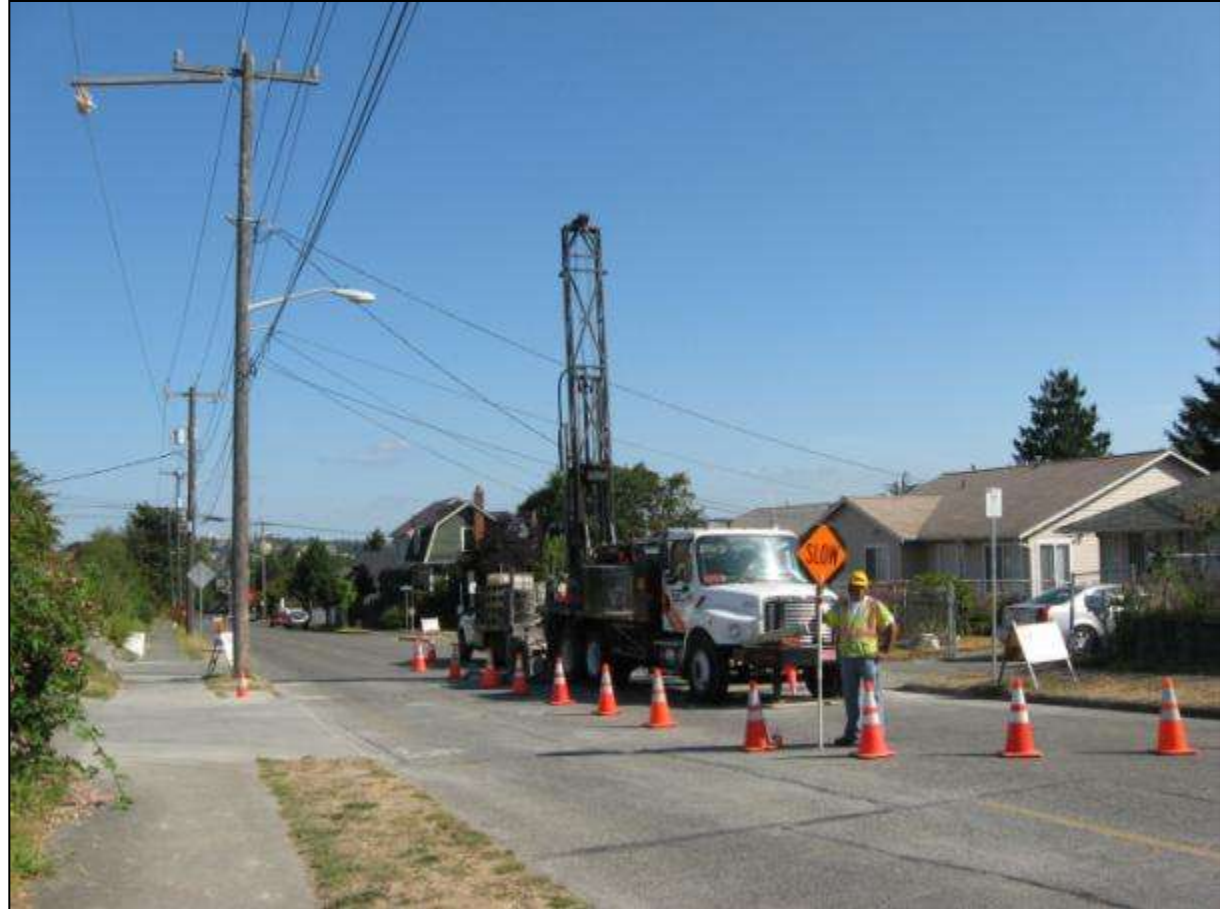
Early phase borings were completed Fall 2011
