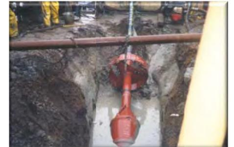
Specific equipment is used for drilling in different conditions. Both drill bits and reaming heads for the Magnolia Project will be selected based on the soil types found at the drill depth
