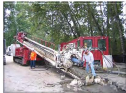
Horizontal Directional Drilling (HDD) Rig used for Drilling and Reaming
