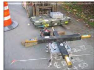
Tracking devices at the surface track the drill bit location during the initial bore
