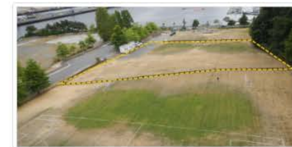
Click image for larger image In December 2017, crews began staging in Smith Cove Park. Equipment is staged within a fence along the yellow, dotted lines..
