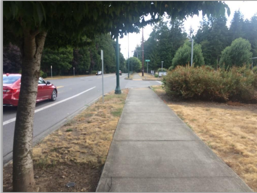
21. Looking south along west side of 244 th Avenue NE just south of Rachel Carson Elementary School midblock crossing. Conditions: 6 feet sidewalk, 5 feet planter, 5 feet paved shoulder.
