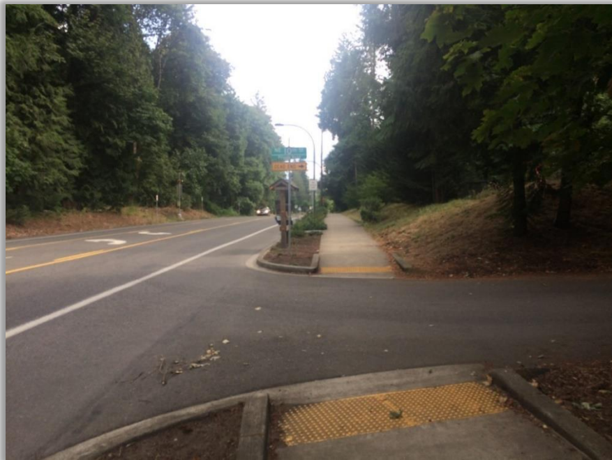
24. Looking south on northwest corner of 244 th Avenue NE and NE 10 th Street. Conditions: 16 feet roadway across NE 10 th Street, 6 feet sidewalk, 5 feet planter, 6 feet paved shoulder. NE 10 th Street is not stop-controlled.
