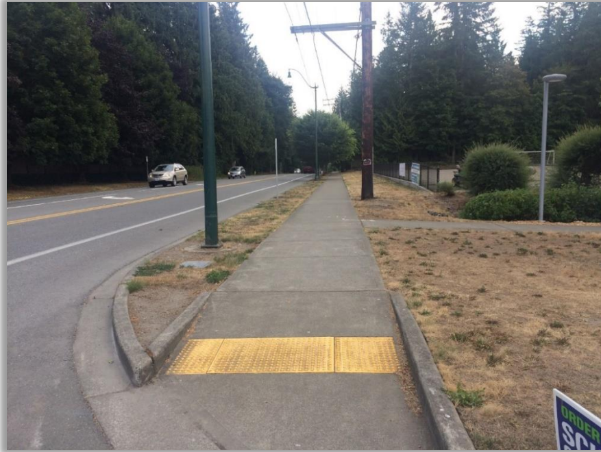
23. Looking south on southwest corner of 244 th Avenue NE and NE 11 th Street. Conditions: 6 feet sidewalk, 5 feet planter, 6 feet paved shoulder.
