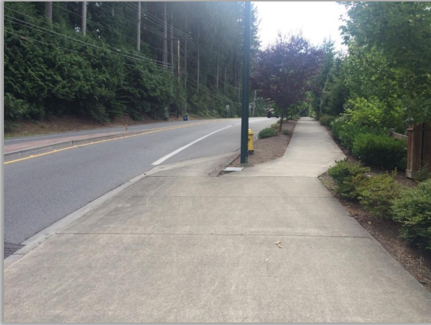
27. Looking west along north side of NE 8 th Street, east of roundabout. Conditions: 12 feet sidewalk transitions to 6 feet sidewalk and 5 feet planter, 10 feet paved shoulder.
