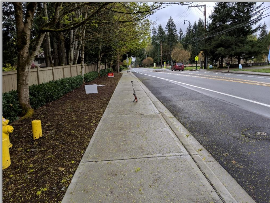
18. Looking south on the east side of 244th Avenue NE approximately 265 feet north of the NE 11 th Street and 244th Avenue NE intersection. Conditions: 6 feet sidewalk, 11 feet paved shoulder transitions to 5 feet paved shoulder.
