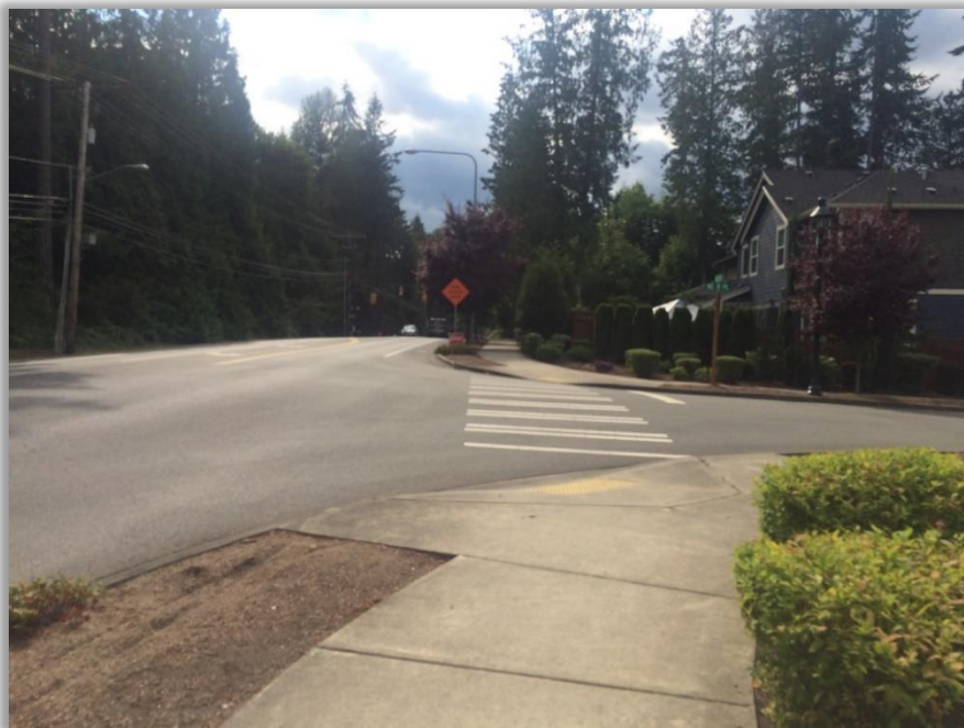
28. Looking west on northeast corner of NE 8 th Street and NE 8 th Place. Conditions: 35 feet roadway across NE 8 th Place, 6 feet sidewalk, 5 feet planter, 6 feet paved shoulder.
