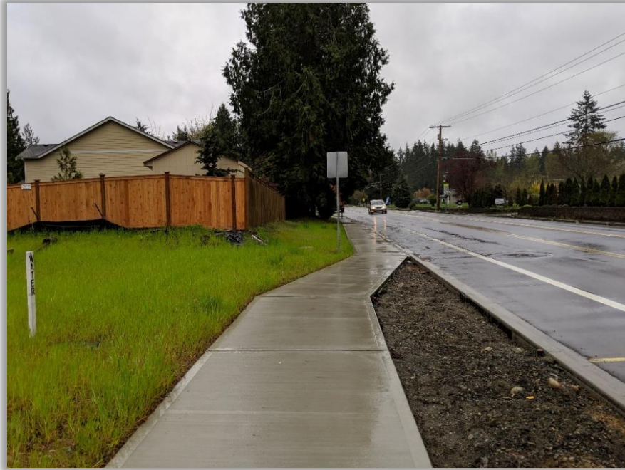
13. Looking south on the east side of 244th Avenue NE approximately 375 feet south of the NE 14 th Street and 244th Avenue NE intersection. Conditions: 6 feet sidewalk and 5 feet planter transitions to 5 feet sidewalk, 6 feet paved shoulder.
