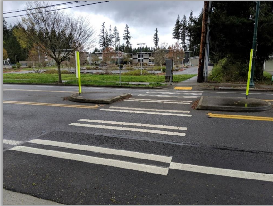
19. Looking west on the east side of 244 th Avenue NE at Rachel Carson Elementary School midblock crossing. Conditions: 41 feet roadway across 244 th Avenue NE.
