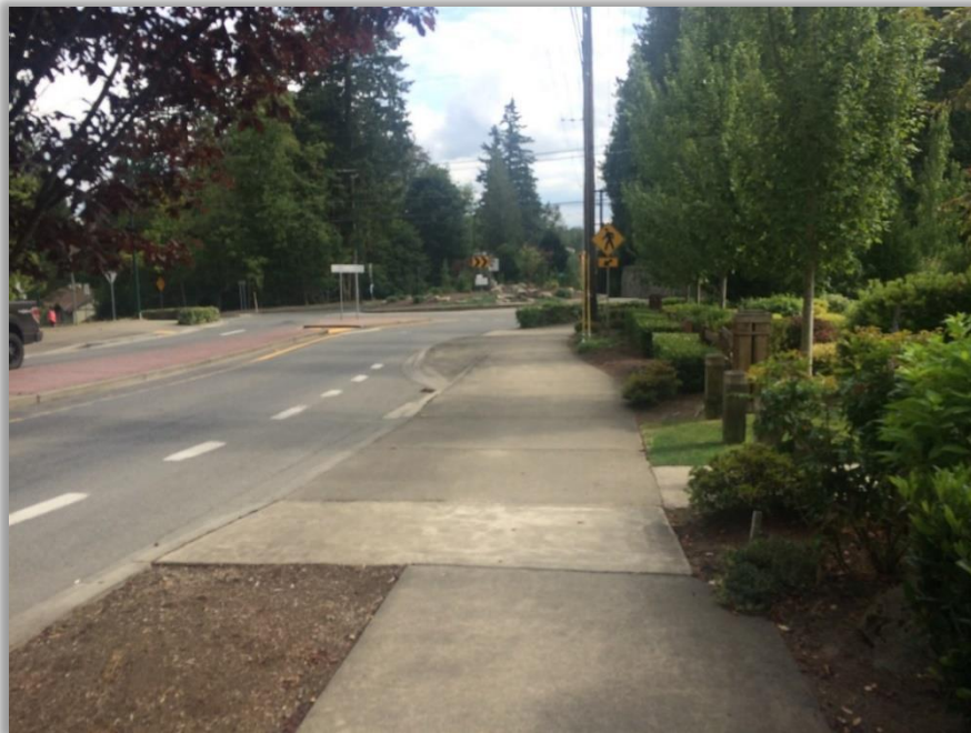
26. Looking south along west side of 244 th Avenue NE approximately 475 feet south of 244 th Avenue NE and NE 10 th Street intersection. Conditions: 6 feet sidewalk and 5 feet planter transitions to 10 feet sidewalk, 5 feet paved shoulder.
