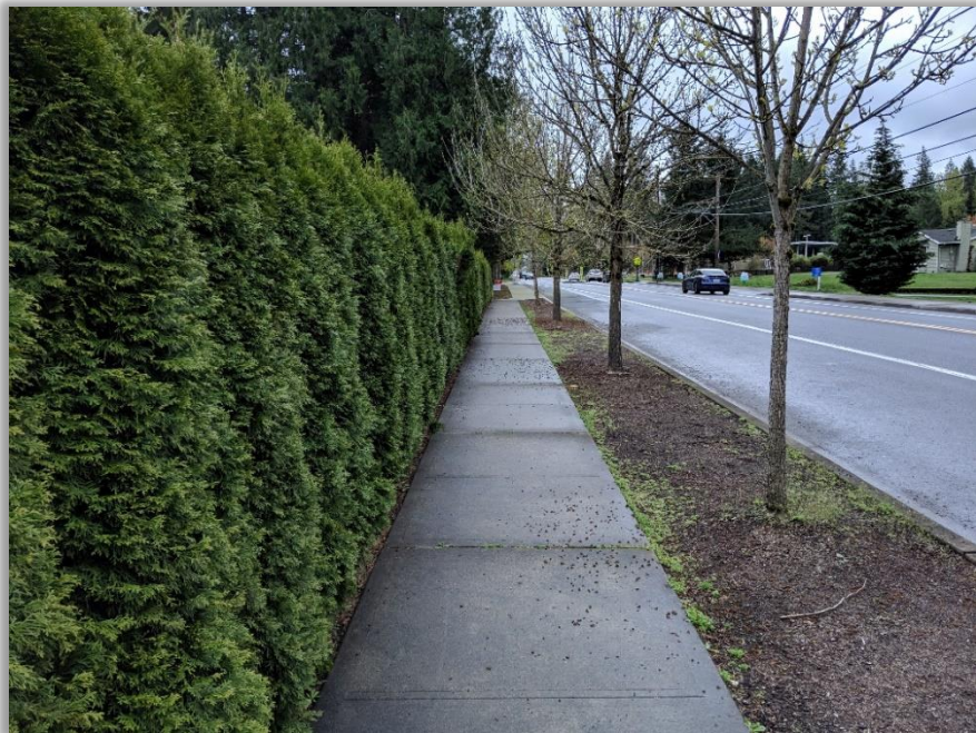
16. Looking south on the east side of 244th Avenue NE approximately 365 feet north of the NE 11 th Street and 244th Avenue NE intersection. Conditions: 5 feet sidewalk and 5 feet planter, 11 feet paved shoulder.
