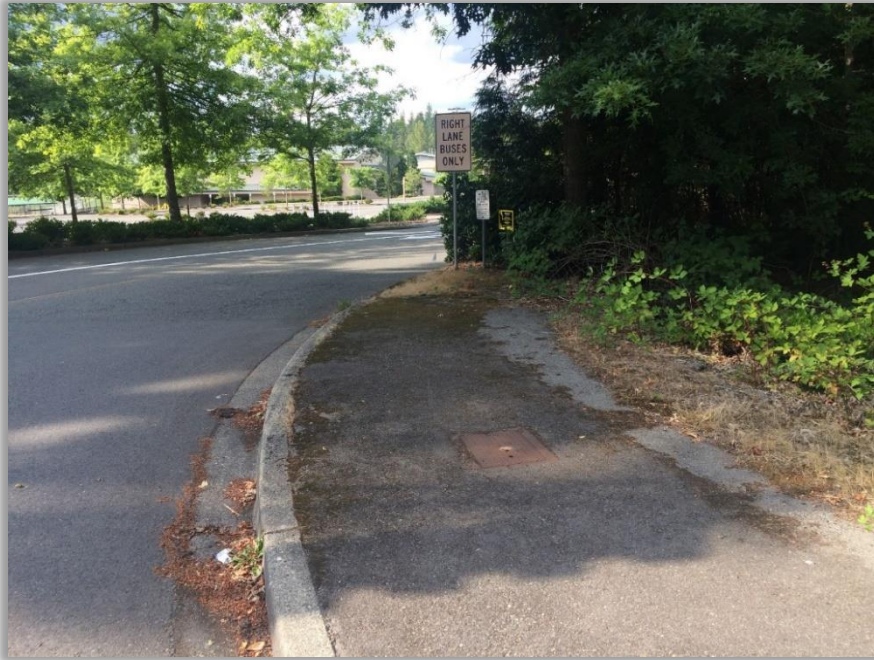
31. Looking north on northeast corner of NE 8 th Street and 242 nd Avenue NE. Conditions: 6 feet asphalt sidewalk.
