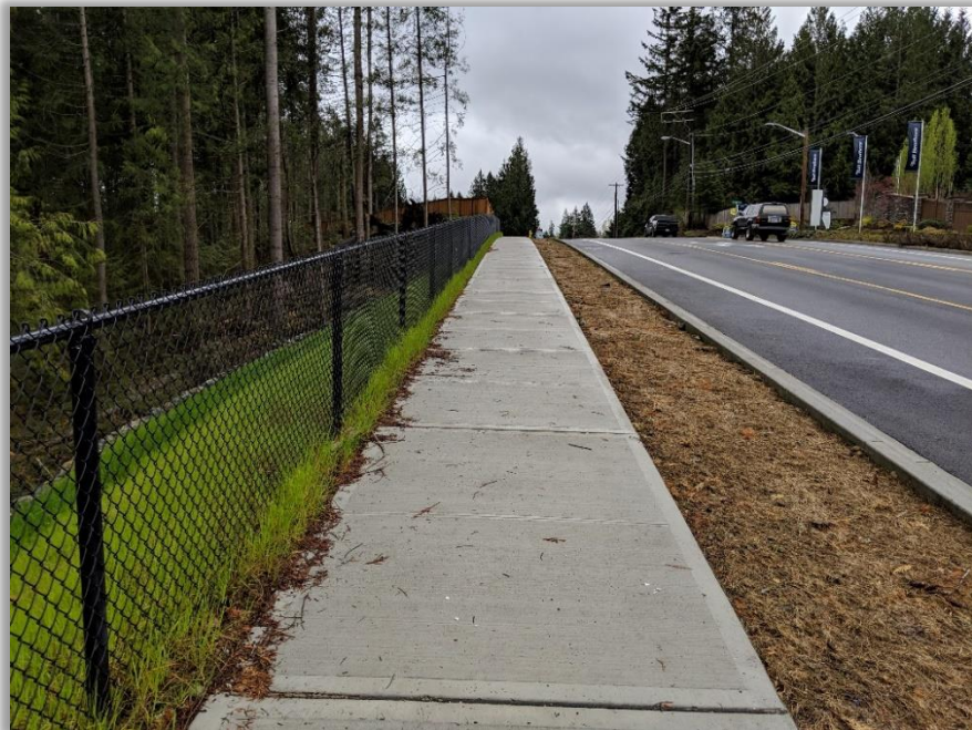
12. Looking south on the east side of 244th Avenue NE approximately 140 feet north of the NE 14 th Street and 244th Avenue NE intersection. Conditions: 6 feet sidewalk and 5 feet planter, 6 feet paved shoulder.
