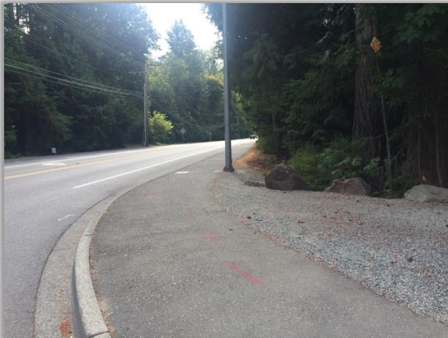
32. Looking west on northwest corner of NE 8 th Street and 242 nd Avenue NE. Conditions: 6 feet asphalt sidewalk, 6 feet paved shoulder.
