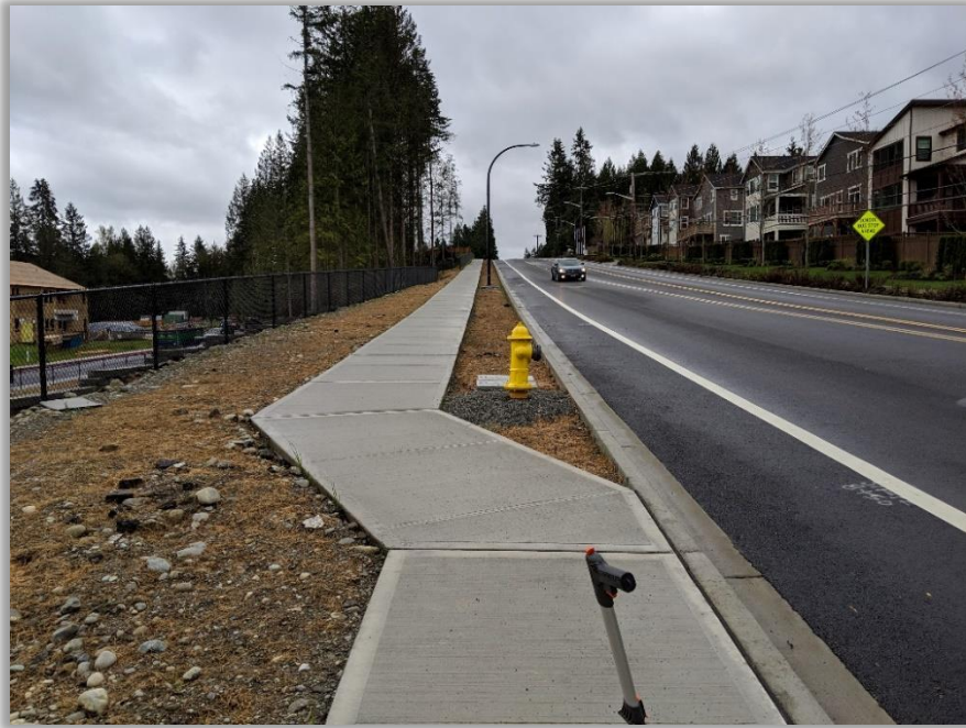
11. Looking south on the east side of 244th Avenue NE at the southeast corner of the NE 16 th Street and 244th Avenue NE intersection. Conditions: 5 feet sidewalk transitions to 6 feet sidewalk and 5 feet planter, 6 feet paved shoulder.
