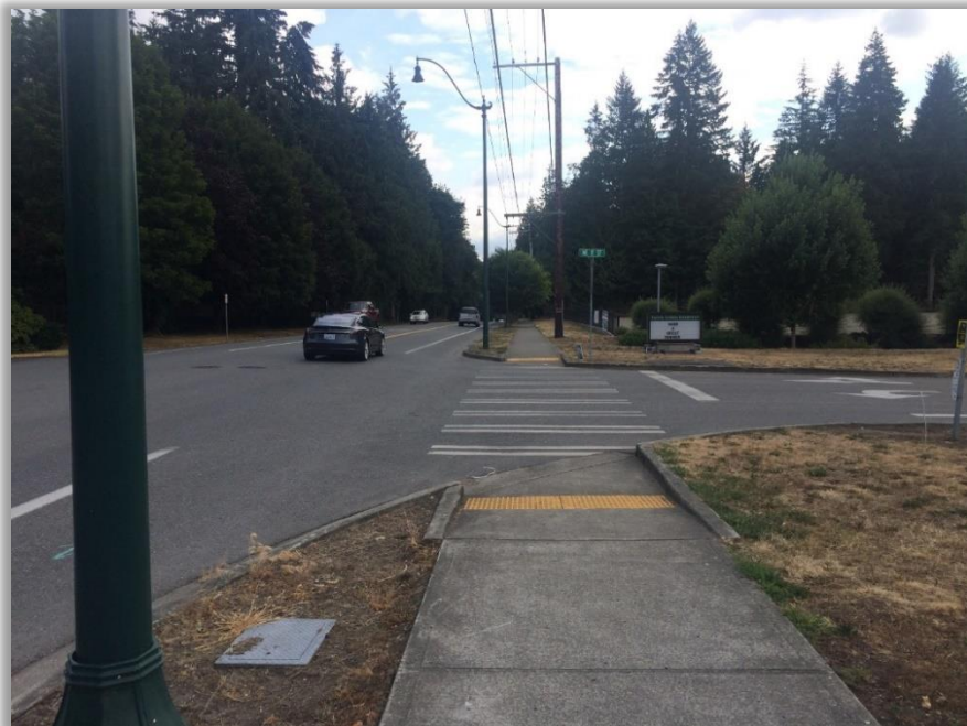
22. Looking south on northwest corner of 244 th Avenue NE and NE 11 th Street. Conditions: 46 feet across Elementary School driveway, 6 feet sidewalk, 5 feet planter, 6 feet paved shoulder. Elementary school driveway is stop-controlled.
