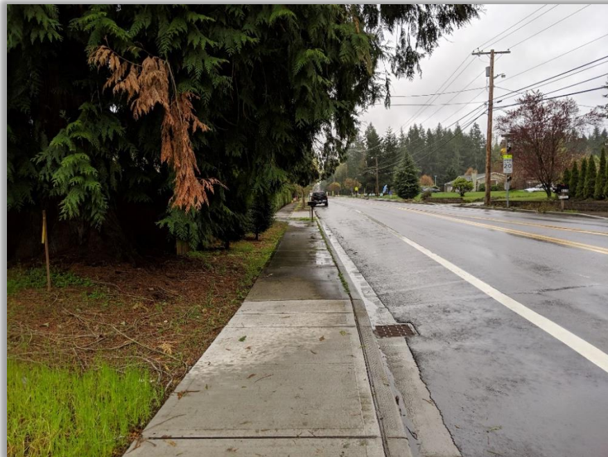
14. Looking south on the east side of 244th Avenue NE approximately 430 feet south of the NE 14 th Street and 244th Avenue NE intersection. Conditions: 5 feet sidewalk and 6 feet shoulder transitions to 5 feet sidewalk and 11 feet paved shoulder.
