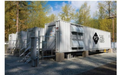
Glacier Battery Storage Installed 2015-2016 2 MW / 4.4MWh
