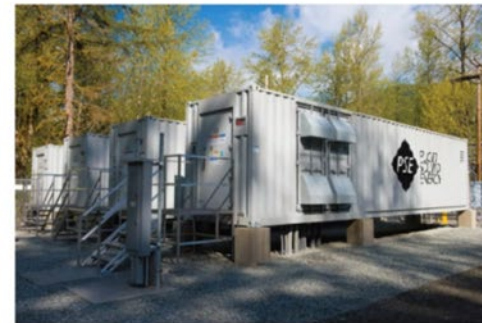
Glacier Battery Storage Installed 2015-2016 2 MW / 4.4MWh
