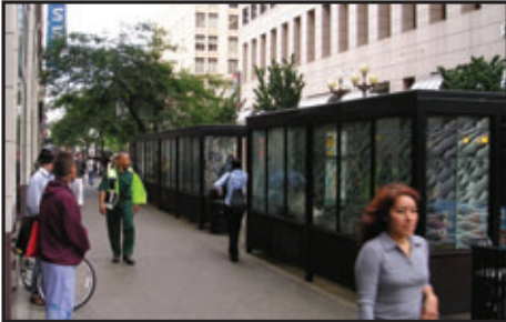
The revamped bus waiting area (top) at Fourth Avenue and Pike Street in downtown Seattle has a more open feel, and more features for safety and access, than the old bus shelters (bottom).
