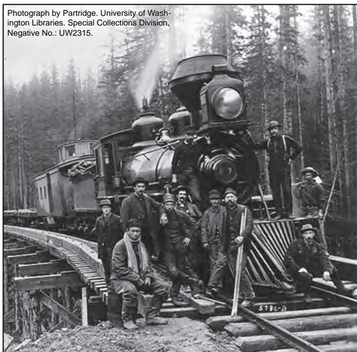
Figure 4-27. Chinese worker (front left) on the Green River Northern Pacific branch line, ca. 1885.
