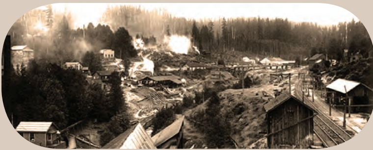
Figure 5-44. The Seattle Coal Mine was at Newcastle, shown here with the New Castle Mine in 1909 (Photograph by Asahel Curtis. University of Washington Libraries, Special Collections, Order No.: CUR622).
