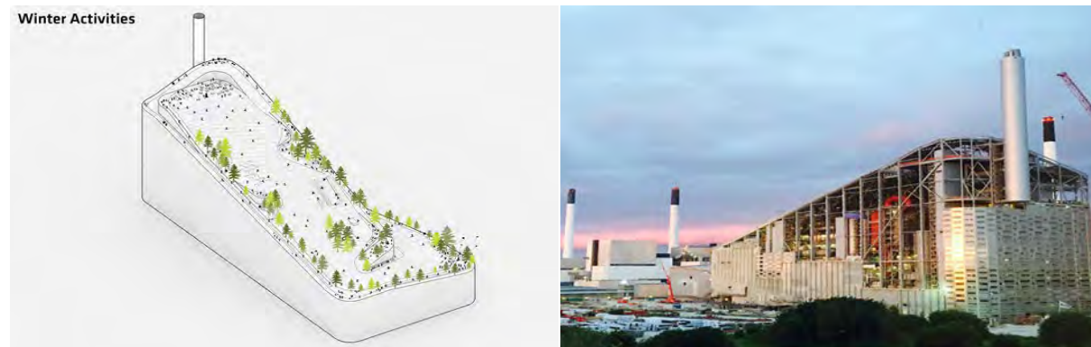
Figure 2–14. Copenhill WTE: Located in Downtown Copenhagen with Recreational Ski Slope and Hiking Trail over the Facility
