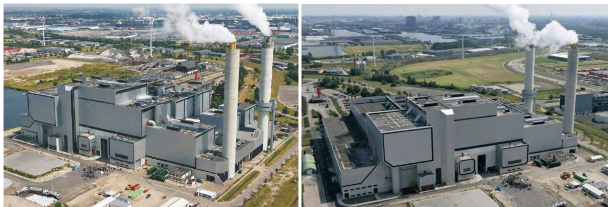
Figure 2–26. WTE Facility in Amsterdam, Netherlands
