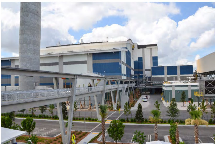
Figure 2–17. Elevated Walkway from Education Center to WTE Facility
