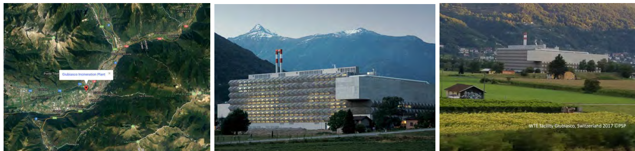
Figure 2–25. WTE Facility in Giubiasco, Switzerland
