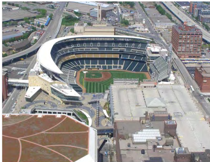
Figure 2–13. Hennepin County, Minnesota: WTE Plant Located in Downtown Area (Background) Adjacent to Target Field Baseball Stadium
