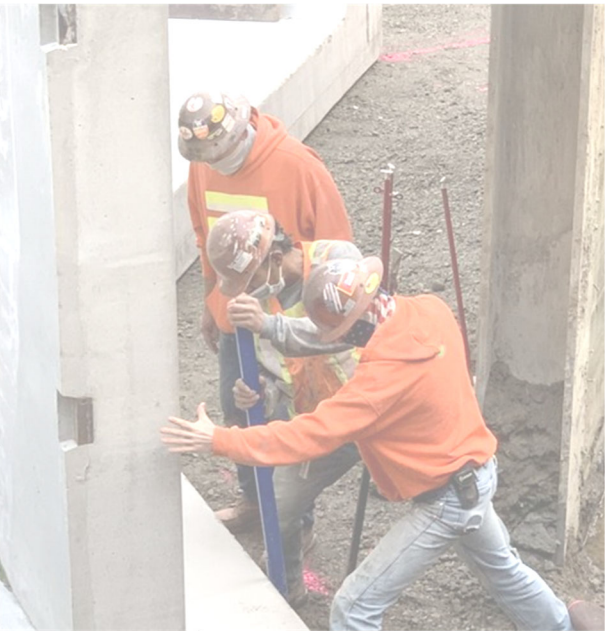
Installing culvert wall at Madsen Creek
