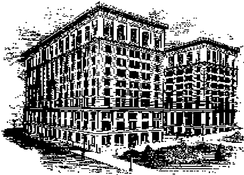
COUNTY - CITY BUILDING---1931
