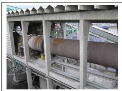
A portion of the 540 ft. long wet process kiln at Lafarge Seattle, formerly the Ideal/Holnam Cement plant. (pavementinteractive.org)
