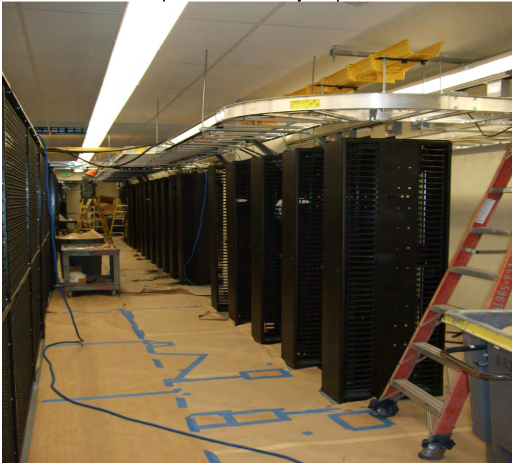
Main Distribution Frame Area - King County Data Center
