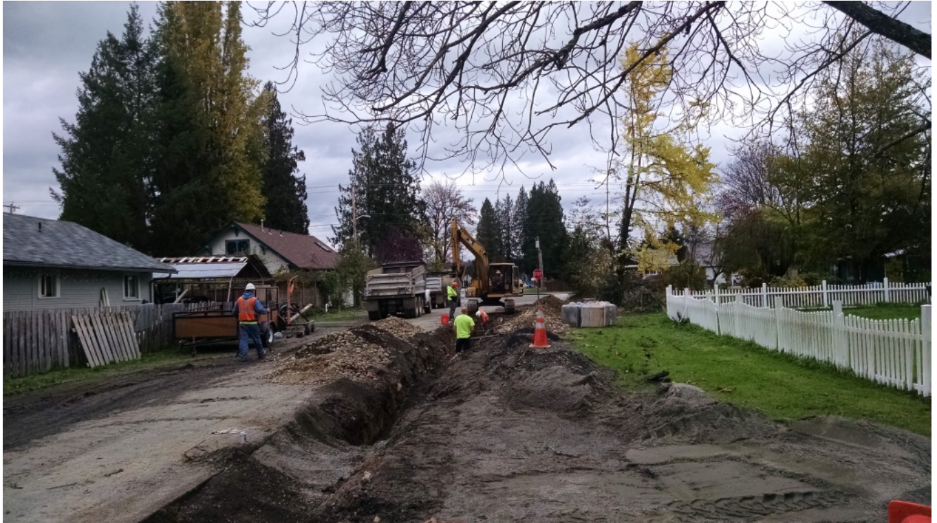
Carnation Water Main Replacement
