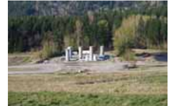
40-foot-high gas flares with buffer zone trees in background.
