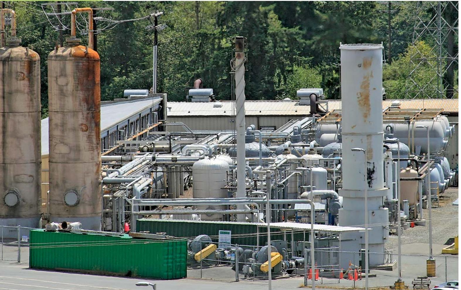
Landfill gas is transported via pipeline from the disposal areas of the Cedar Hills Regional Landfill to the onsite BioEnergy Washington plant. Once there, the gas is converted into renewable natural gas.
