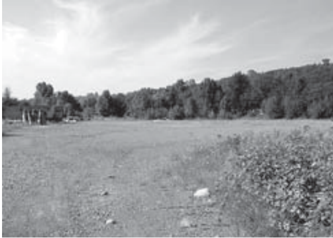
▲ South Park Landfill, one of the closed landfills managed by King County
