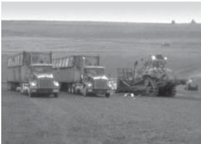
▲ Area 5 of the Cedar Hills Regional Landfill
