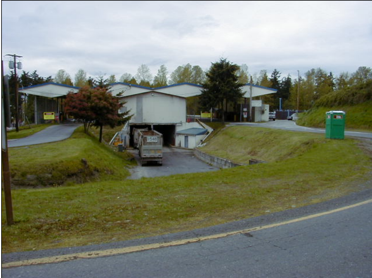
The old style partial end walls leave the facility open to the elements.
