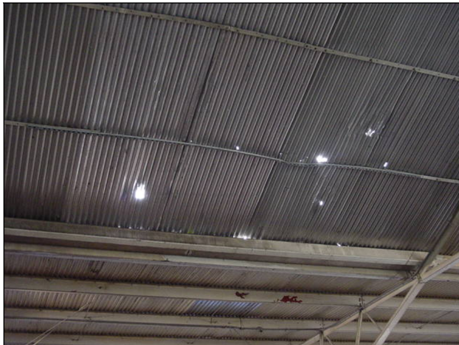
Roof damage caused by a collection vehicle.
