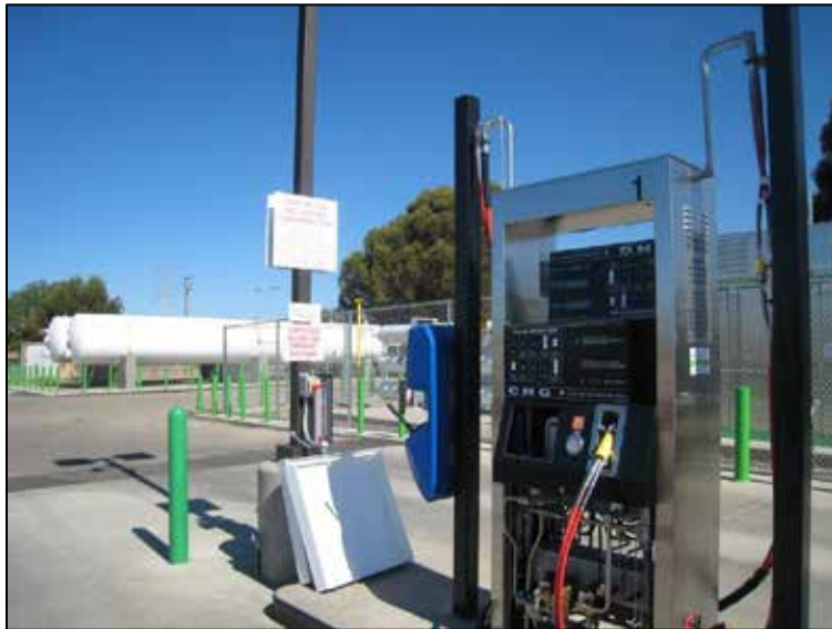
Figure 3-16. CNG Fueling Station from Biogas Produced at the Clean World Anaerobic Digestion Facility in Sacramento California
