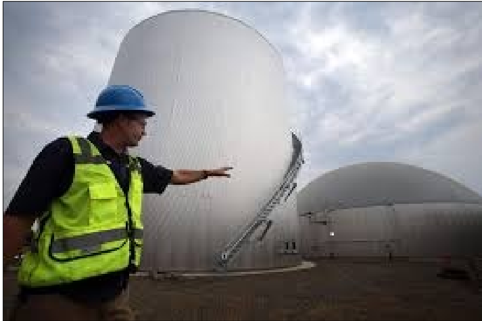
Figure 3-18. JC-Biomethane’s Anaerobic Digestion Facility in Junction City, Oregon
