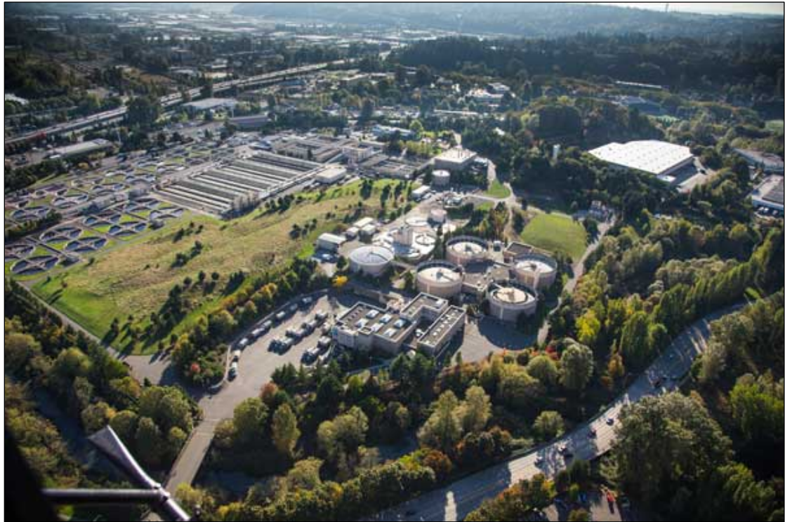
Figure 4-2. Renton Wastewater Treatment Plant
