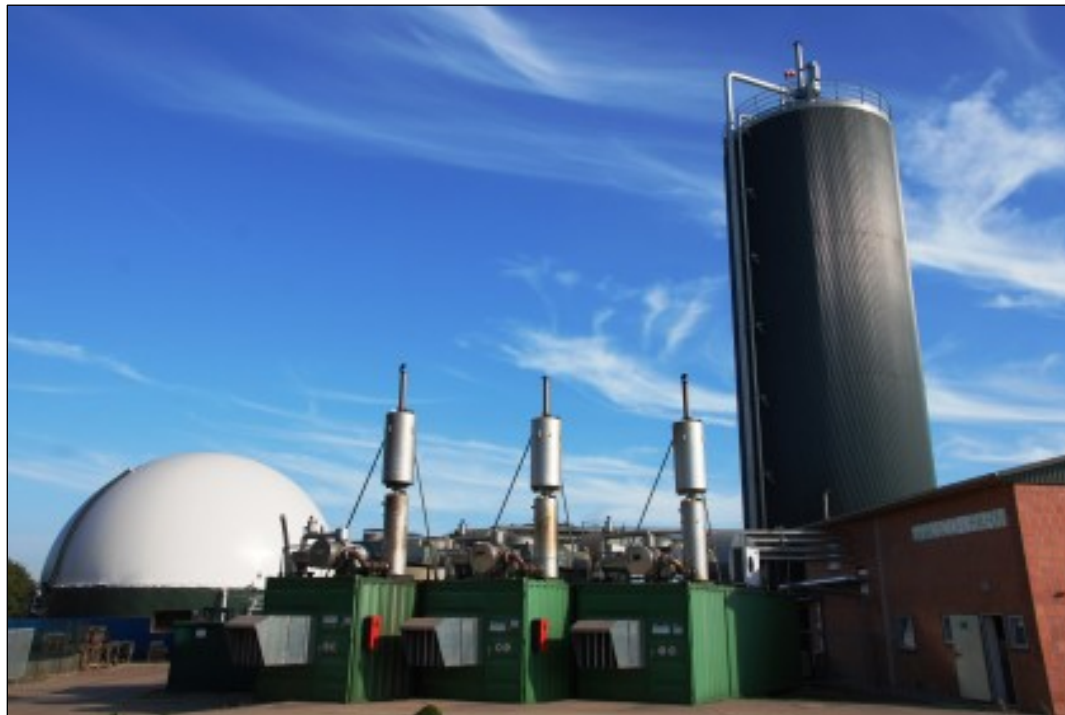
Figure 3-20. Vertical Plug Flow Digester
