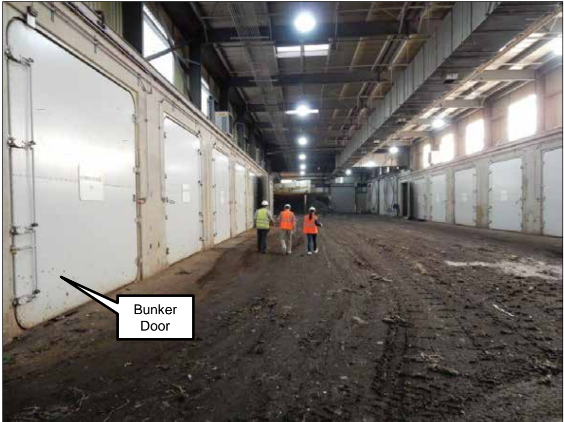
Figure 3-23. ZWED Dry Fermentation Facility Bunkers in San Jose, California
