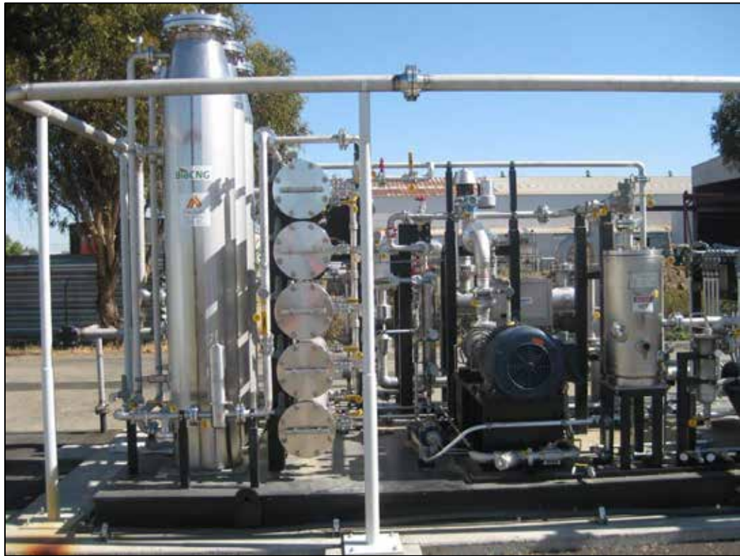
Figure 3-17. Biogas Upgrading System at the Clean World Anaerobic Digestion Facility in Sacramento, California
