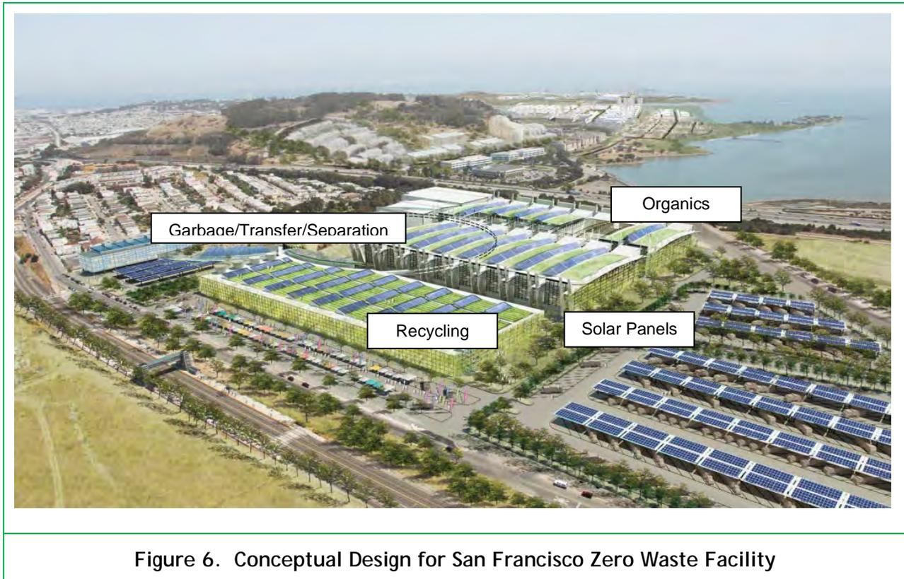
Figure 6. Conceptual Design for San Francisco Zero Waste Facility
