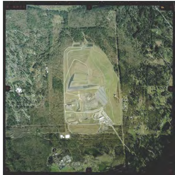
Cedar Hills Landfill currently operates with a 1,000 foot buffer leaving up to 900 feet of usable space.
