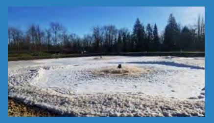
Water that seeps through garbage (leachate) is piped to the leachate lagoons, aerated, then piped to a <u>wastewater</u> facility
