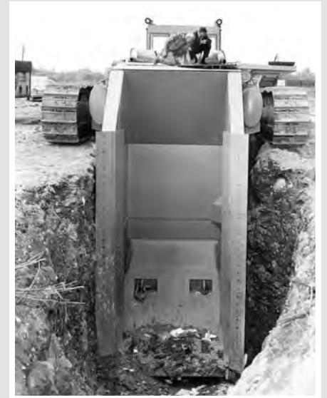
A 350,000 pound piece of landfill equipment called the "Mole" is used to compact solid waste dumped into trenches.
