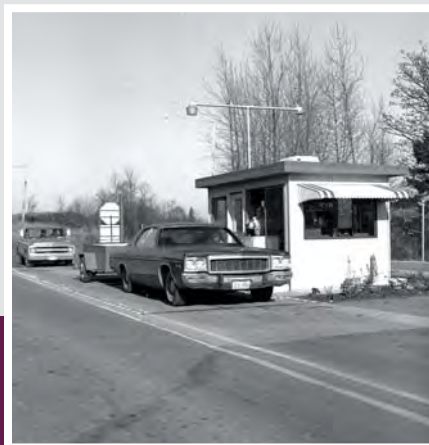
Scales and a scale house are also installed in the late 1970s. Vehicles weigh in at the scale house to provide an accounting of the tons of waste disposed at the landfill each year.
