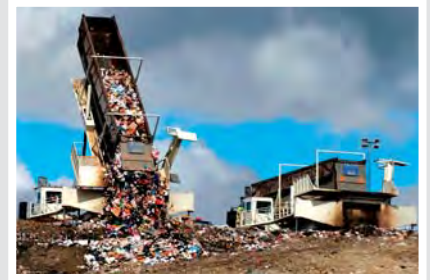
In 2008, tippers are used to empty trailers, replacing the walking floor trailers previously used. The tippers save staff time and other resources, as well as reduce equipment damage.
