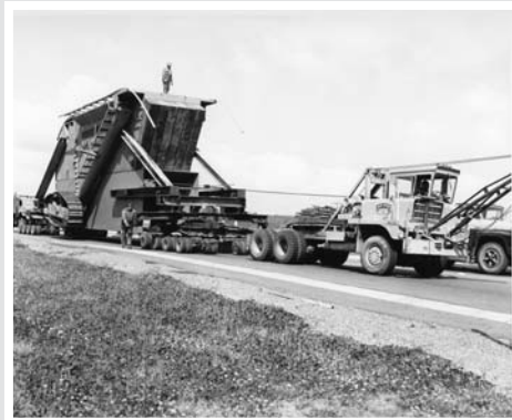
A 350,000 pound piece of landfill equipment called the "Mole" is used to compact solid waste dumped into trenches.
