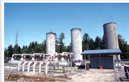
Landfill gas is generated as the buried waste decomposes. In the 1980s, an extensive gas collection system is installed, routing the gas to high-temperature flares, where it is burned and harmful emissions are safely destroyed. Active gas collection begins in the late 1980s.
