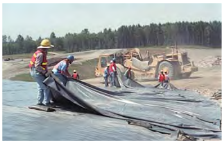
From the mid-1980s to mid-1990s, older areas of the landfill receive cover systems and environmental controls.
