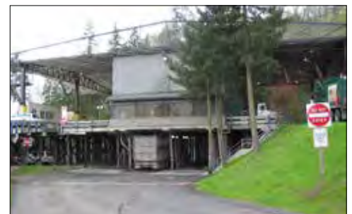
Refuse trailers located below tipping floor
