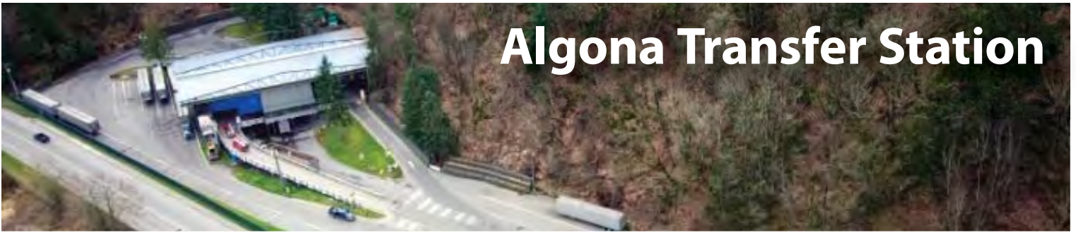
Aerial view of Algona Transfer Station
