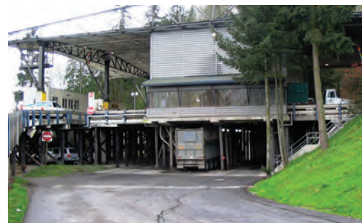
Refuse trailers located below tipping floor.
