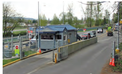
Entrance to the station.
