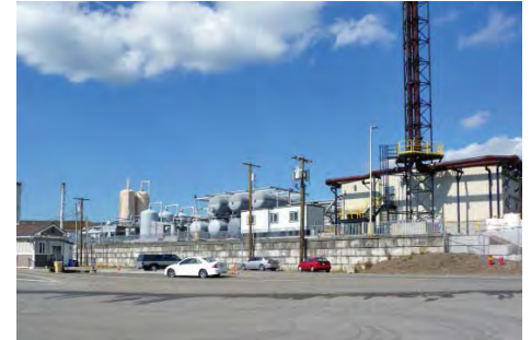
Bio Energy Washington landfill gas-to-energy plant
