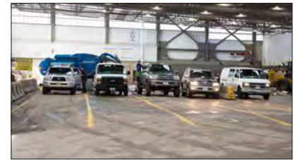
New transfer building has large self-haul customer unloading areas
