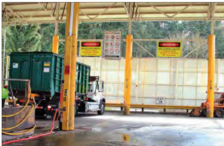
A commercial garage truck on the tipping floor
