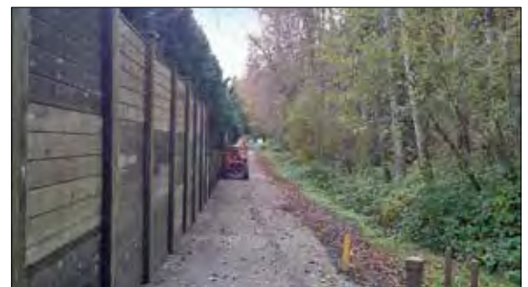
Constructed in 2011, a sound barrier wall along the west side of the transfer station helps reduce noise impact to neighbors
