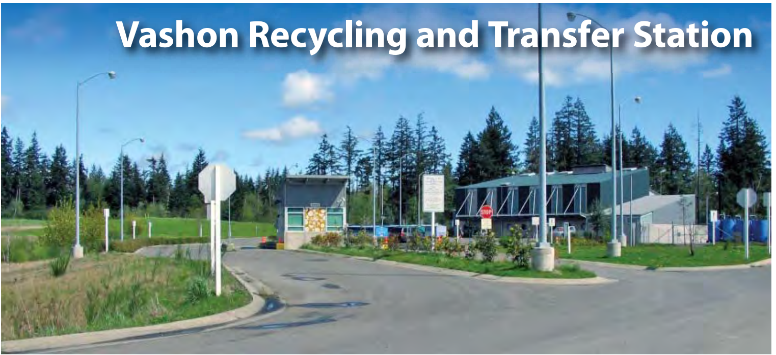
Exit and entrance to scalehouse
