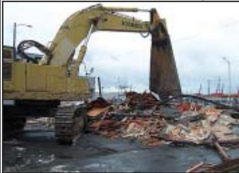
"The Nibbler" at work sorting through demolition debris.
