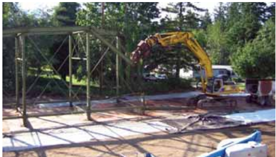
Mt. Si Bridge in North Bend as it is deconstructed.
