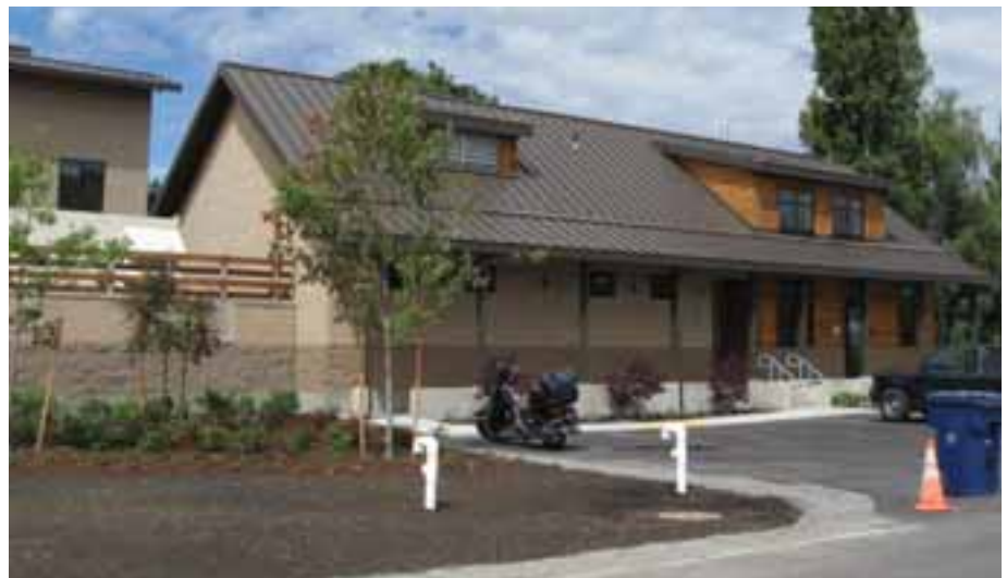
Carnation Treatment Plant Operations and Maintenance building.
