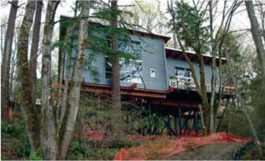
2007 LEED grant recipient Mercer Slough Environmental Education Center. This project also received a 2008 "Excellence in Building Green Award."
