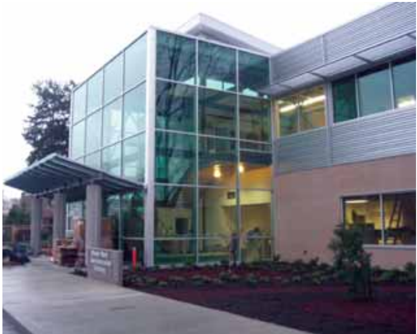
South Treatment Plant Administration Building – Front Entrance During Construction
