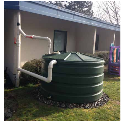
Water cistern to capture runoff from school roof.
