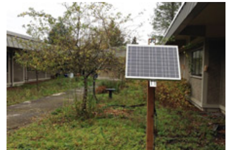
Solar panel powers the cistern pump in the school garden
