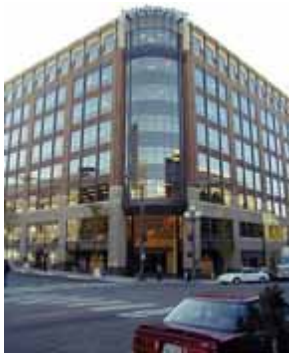
King Street Center's green building features save county money.
