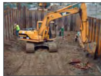
Excavating the area for the pump station.
